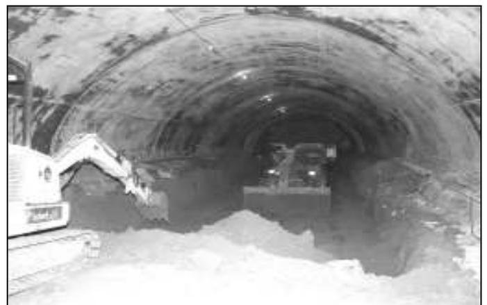
Fig. 3. Belgian tunneling method, Line H, 2000.
