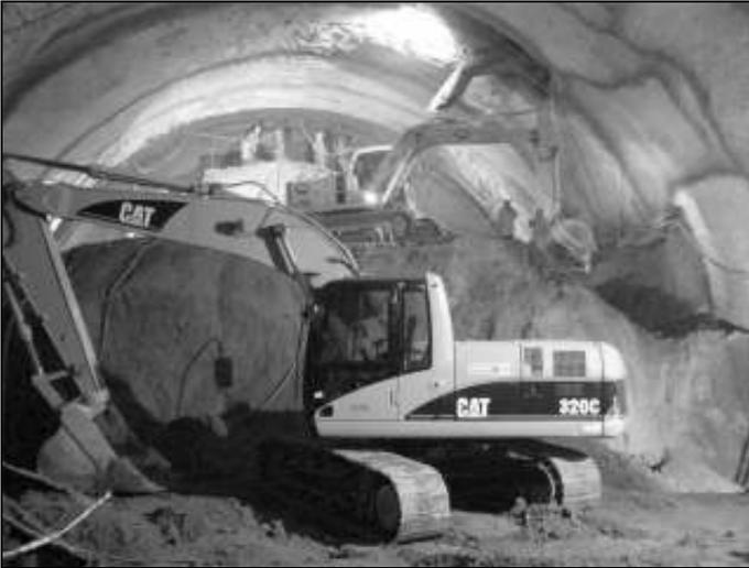
Fig. 9. Corrientes Station, Line H. Full face excavation.
