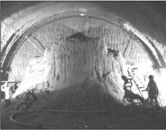
Fig. 4. Full face excavation, Line B, 2004.
