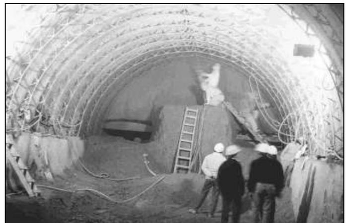
Fig. 2. First use of shotcrete, Line B.
