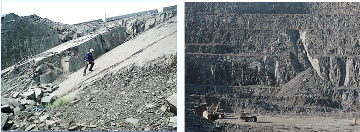
*Figure 1. Flat (left) and wedge (right) failures of rock mass blocks along joints on open pit slopes*
